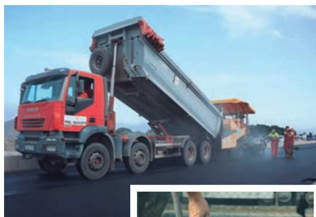
Section of road paved with disused agglomerate by Horinsa
